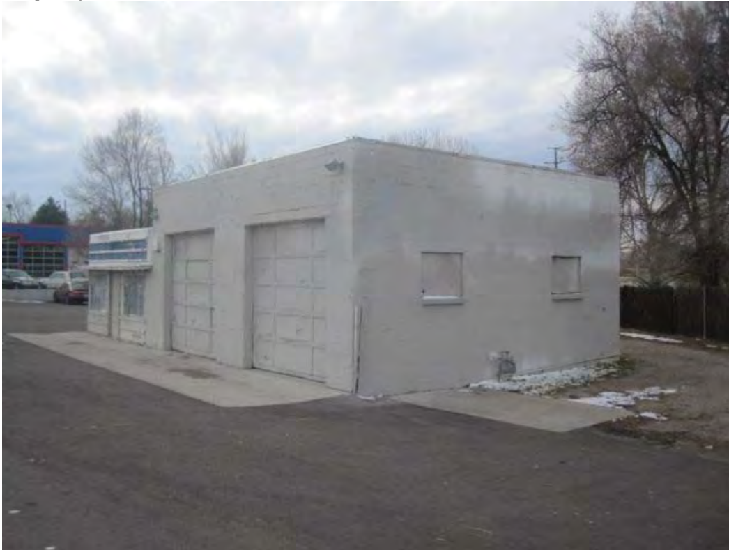
Photo 5DV11363_3 View looking southwest at north and east (front) elevations.
