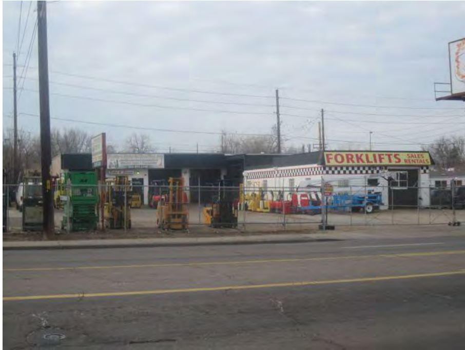
Photograph 2: Western Material Handling (5DVI 1370) View looking northwest
