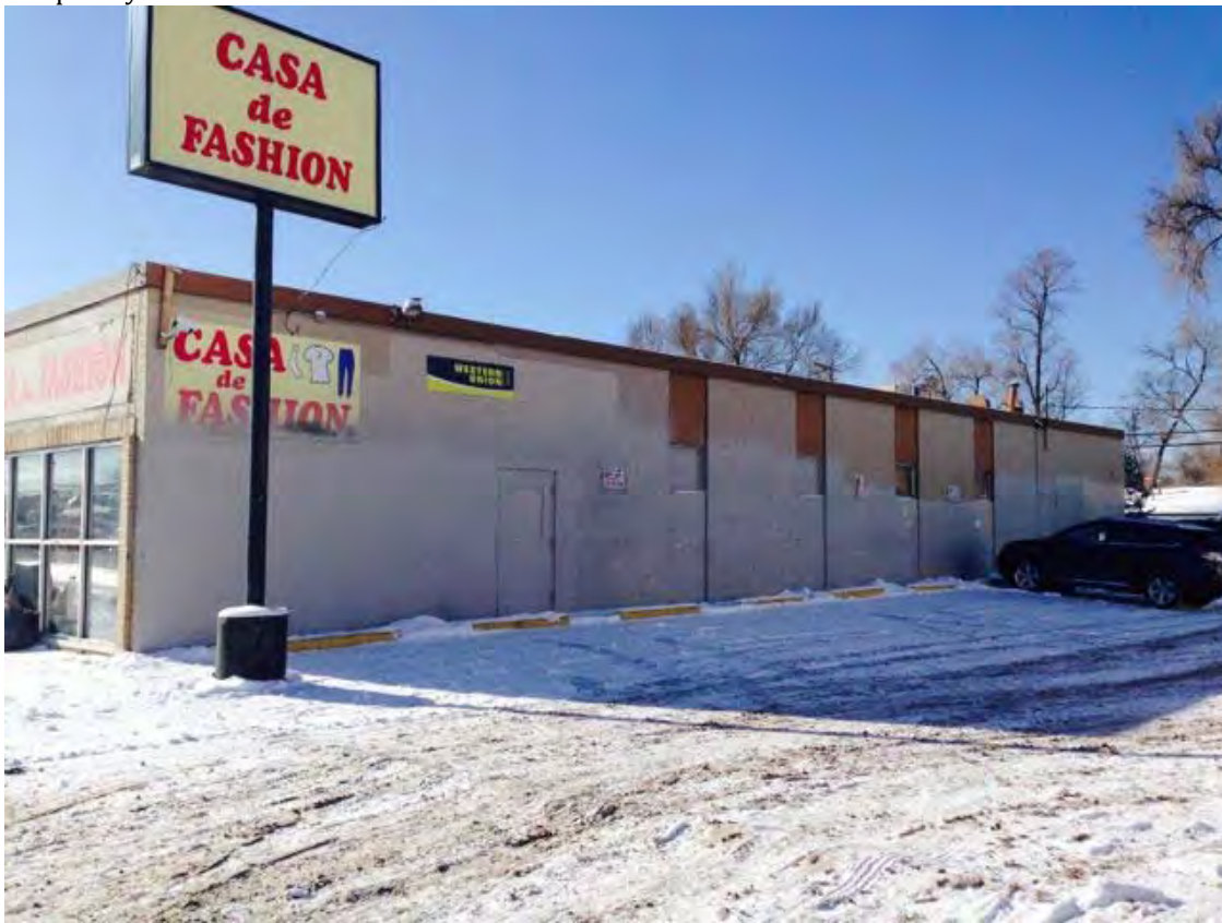
5DV11366_5 View looking southwest at north elevation of 969 Federal Boulevard.
