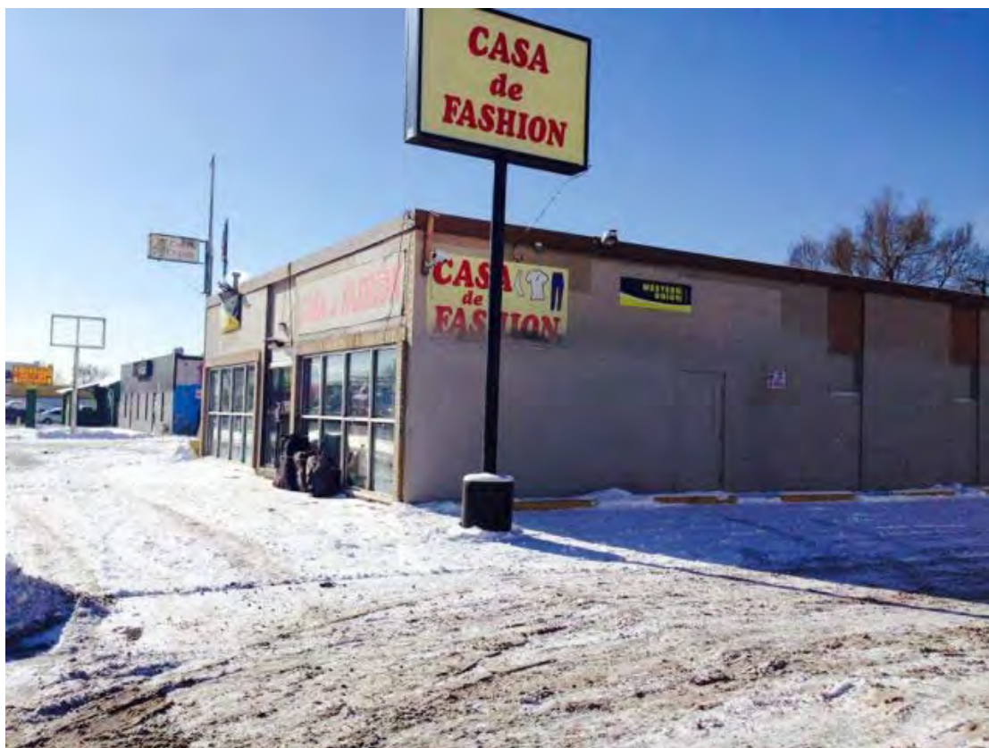
5DV11366_4 View looking southwest at east façade and part of north elevation of 969 Federal Boulevard.
