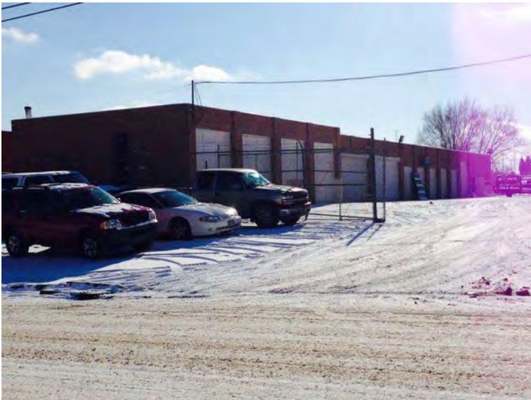
5DV11373_8 Looking southeast at north and west elevations of warehouse with 6-garage bays.
