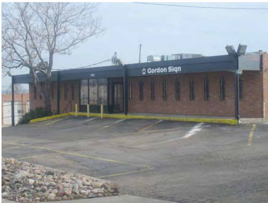
Photograph 12: Gordon Sign (5DVI 1373) Looking southeast at main office building
