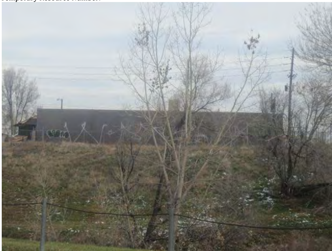
Photo 5DV11372_3 View looking east at west elevation.
