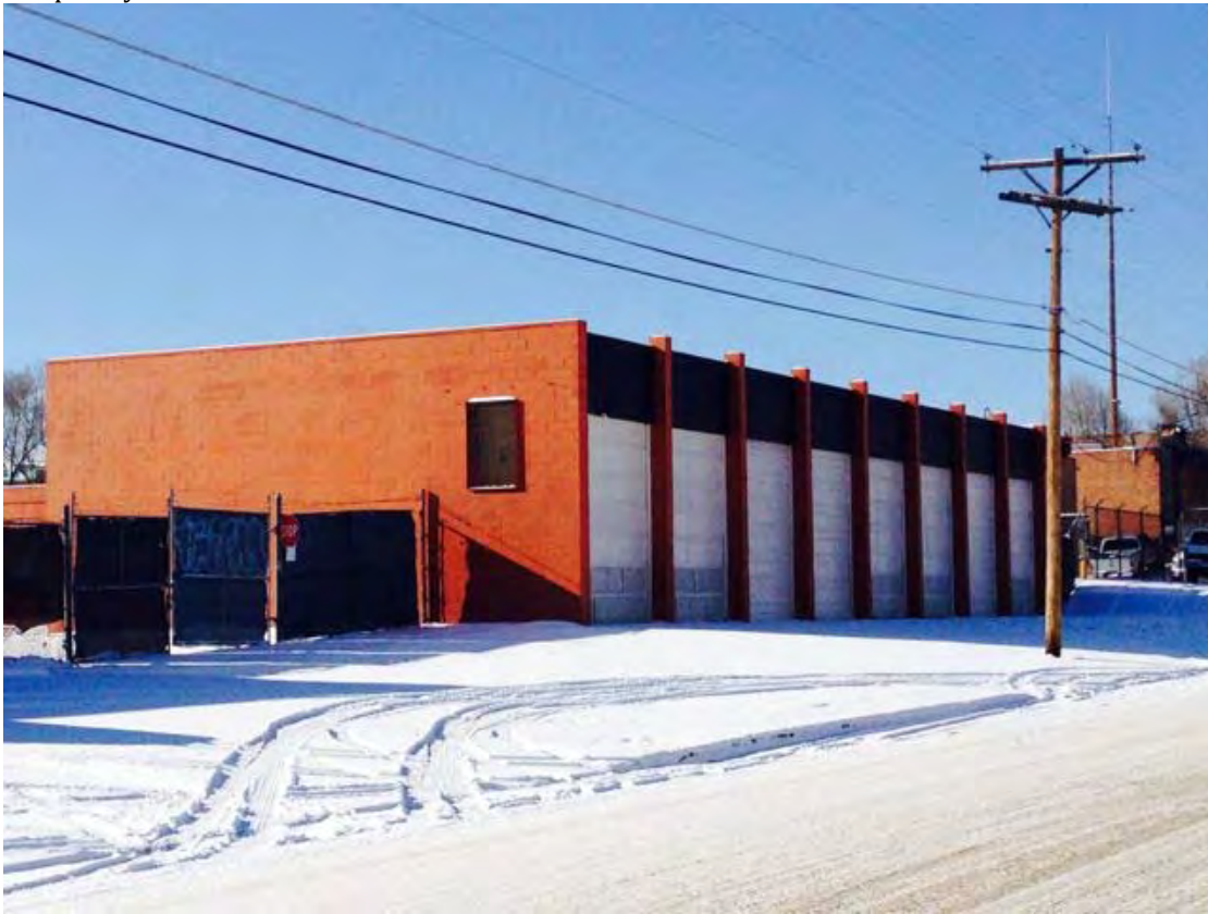
5DV11373_5 View looking southwest at north (front) and east elevations of 8-bay garage building.
