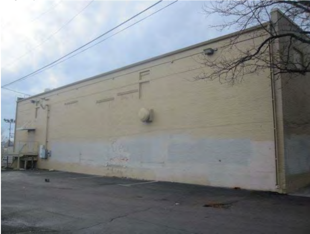
Photo 5DV11365_3 Looking west at east elevation. Note enclosed fenestration.
