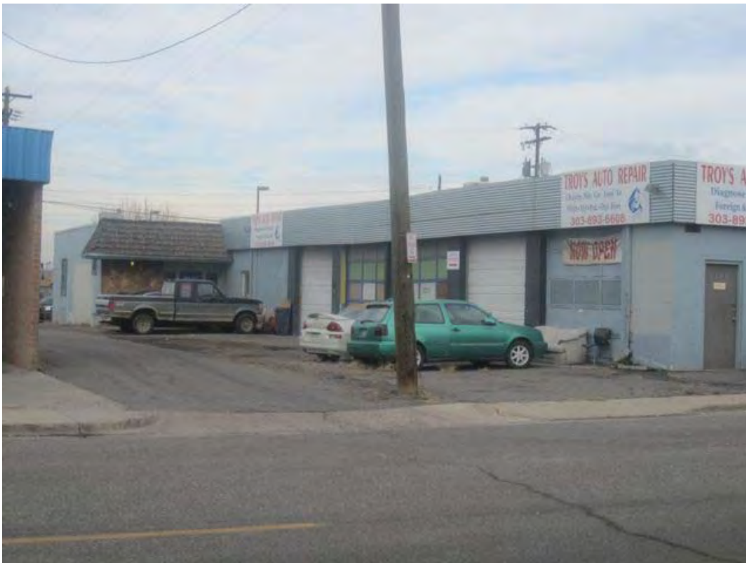
Photo 5DV11400_4 View looking northeast at west elevation.
