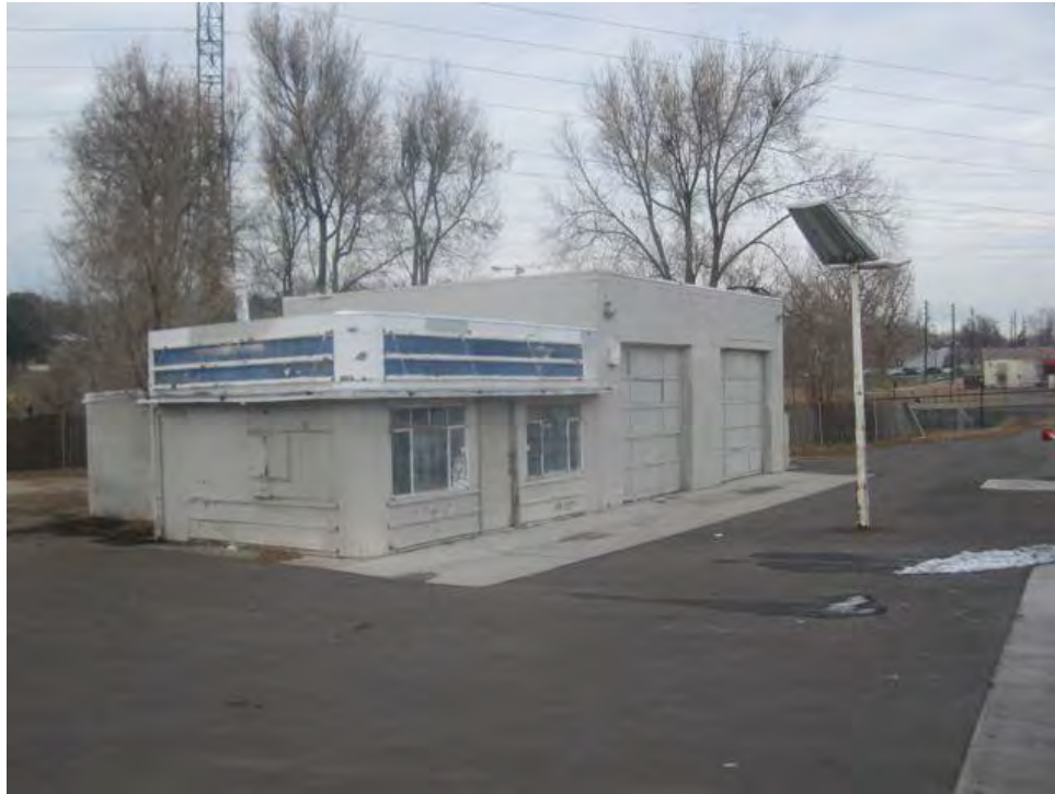
Photograph 9: Vigil's Shamrock Service Station (5DVI 1363) View looking northwest
