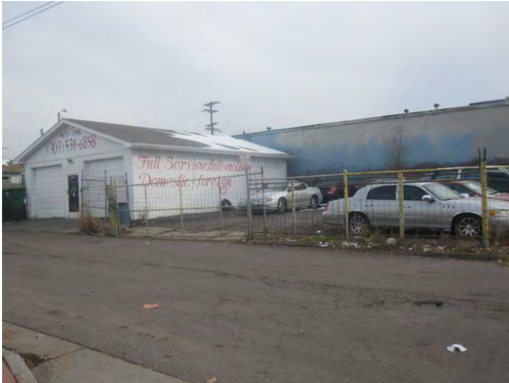
Photograph 10: Complete Auto Care (5DV11371) View looking southeast
