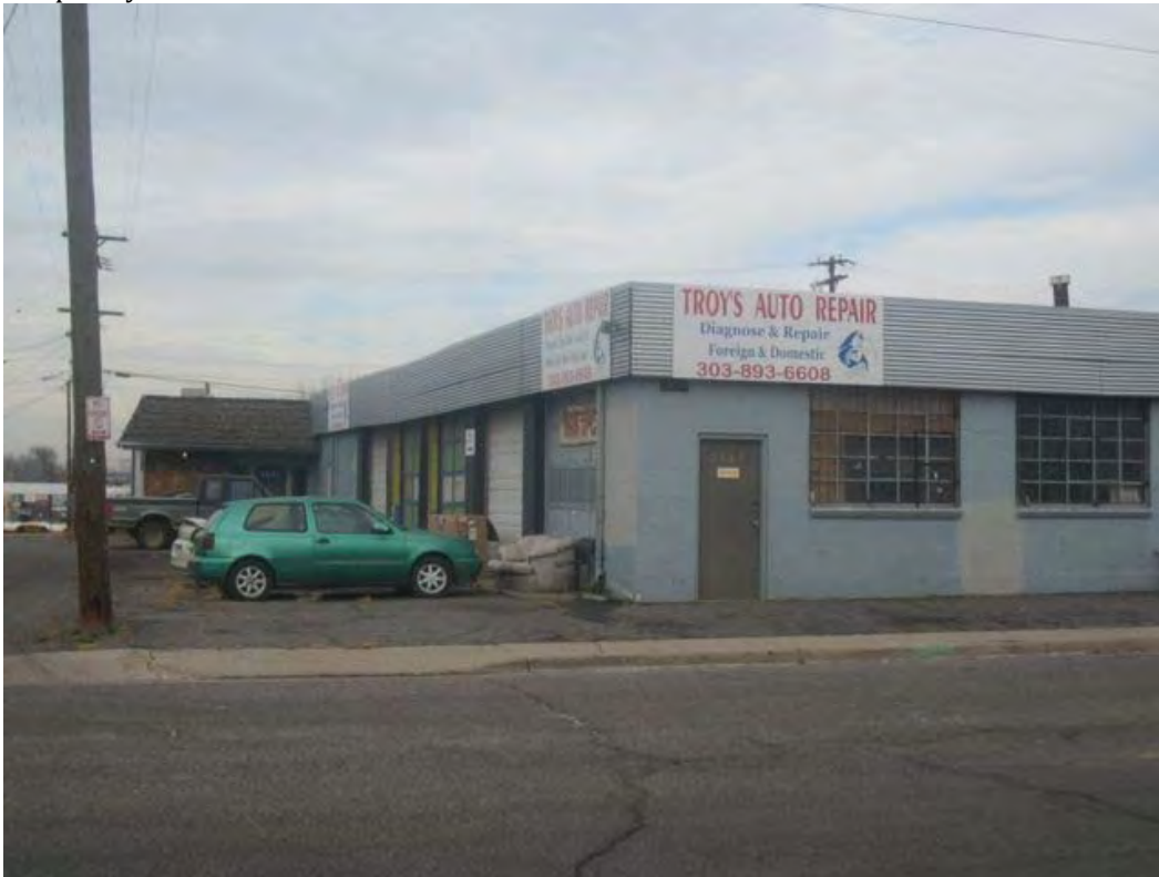
Photo 5DV11400_3 View looking northeast at south (front) and west elevations.
