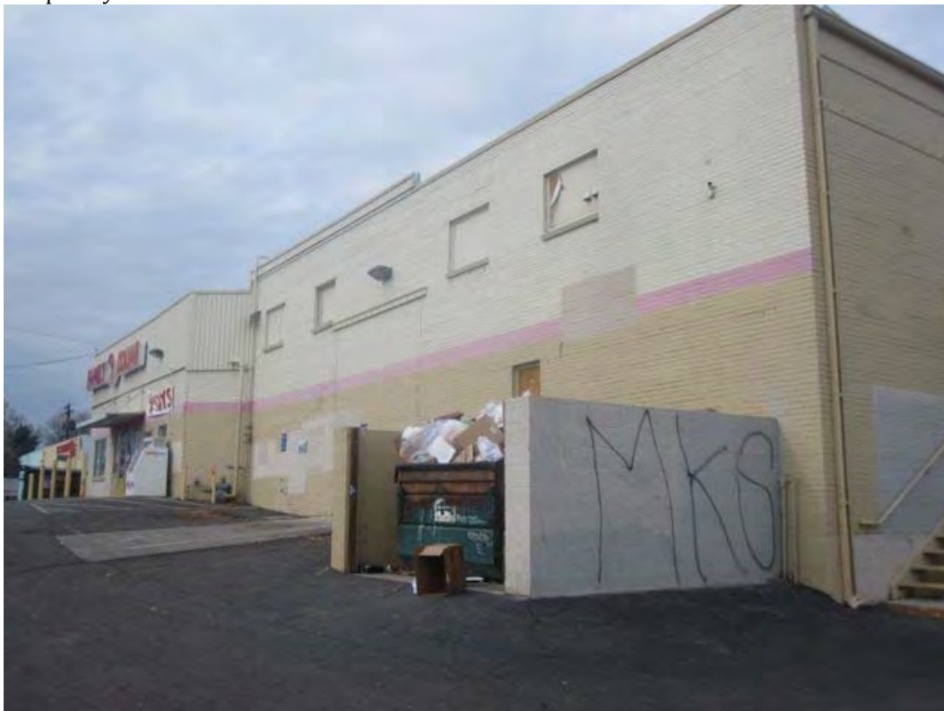
Photo 5DV11365_5 Looking northwest at south elevation.
