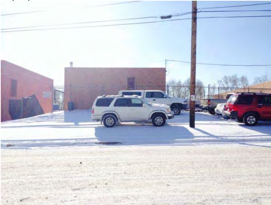
5DV11373_7 Looking south at north elevation of warehouse with 6-garage bays.
