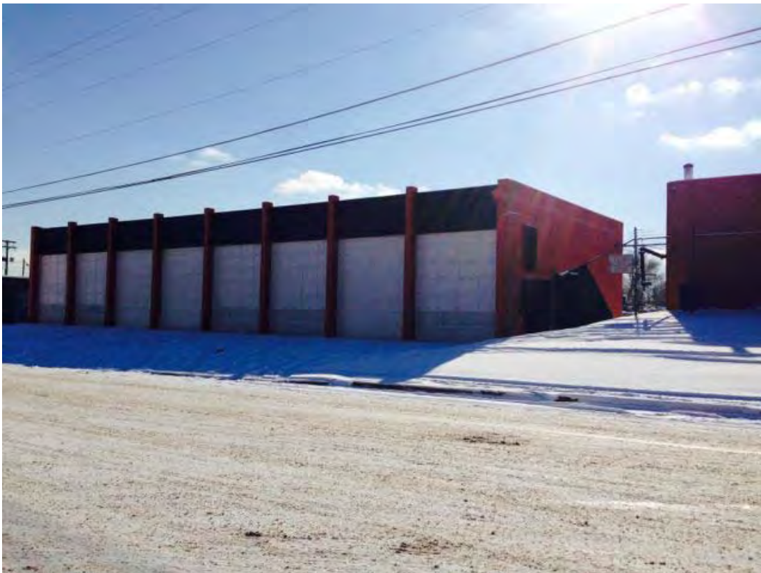
5DV11373_6 View looking southeast at north (front) and west elevations of 8-bay garage building.
