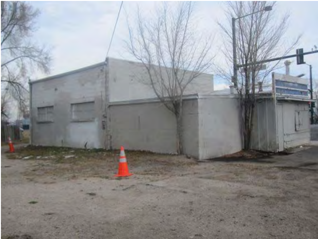
Photo 5DV11363_4 View looking southeast at west (rear) and north elevations.
