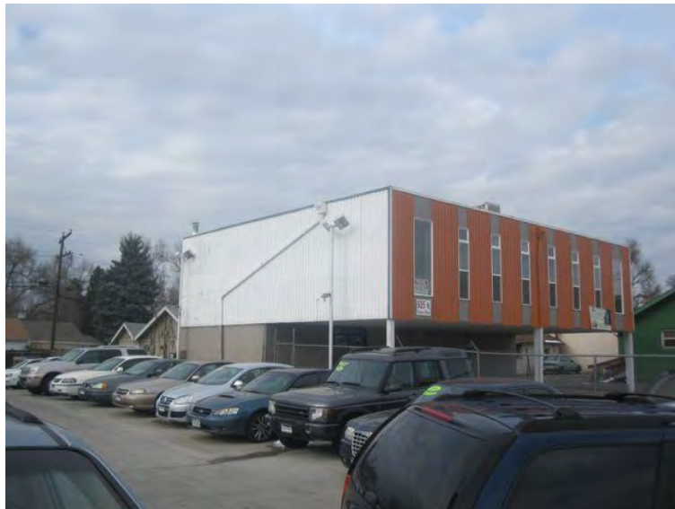
Photograph 4: 913-925 Federal Boulevard (5DVI1368) View looking northwest
