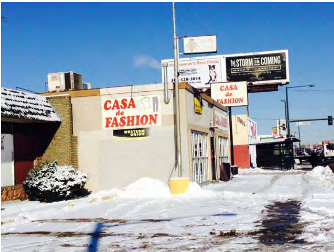
5DV11366_6 View looking northwest at east façade and part of south elevation of 969 Federal Boulevard.
