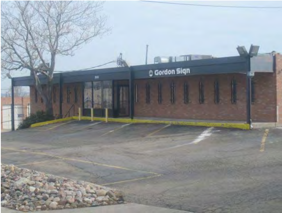
Photo 5DV11373_3 View looking southeast north (front) elevation.
