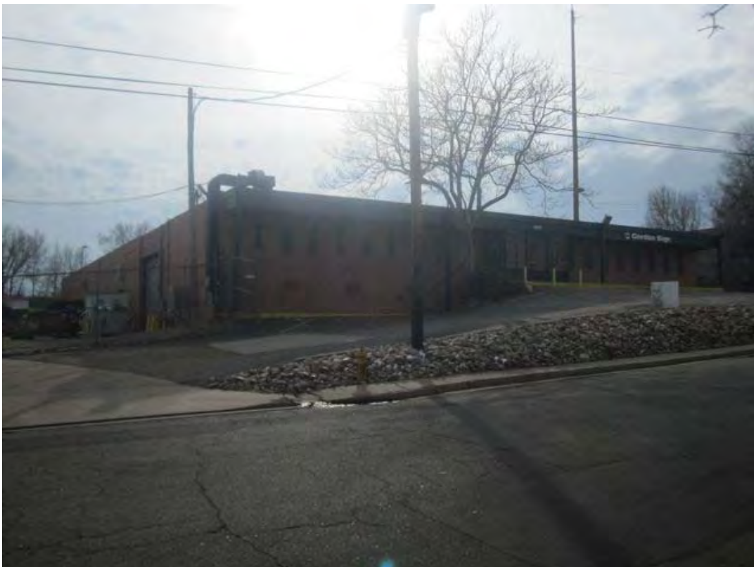
Photo 5DV11373_4 View looking southwest at north (front) east elevations.
